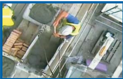
View from Crane Operator's Cab
