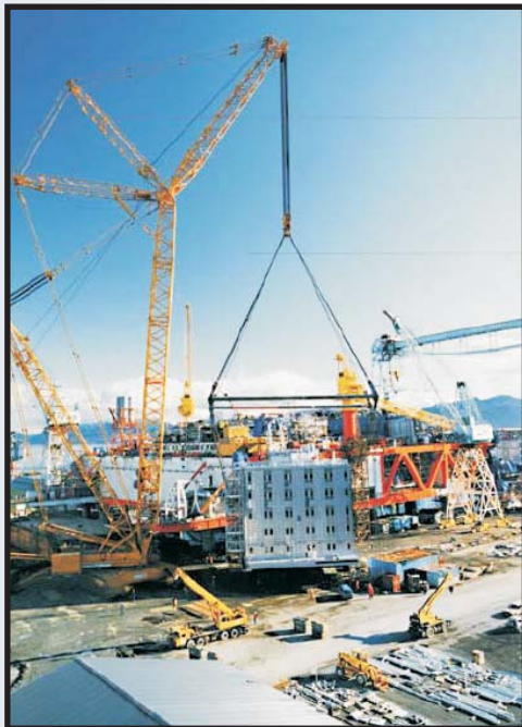
Rigging Pro is an essential tool in all lifts
